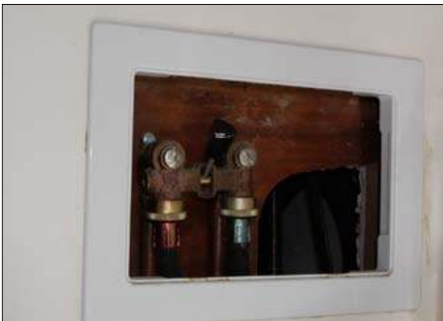
MR124 Single-Throw Clothes Washer Shut-Off
