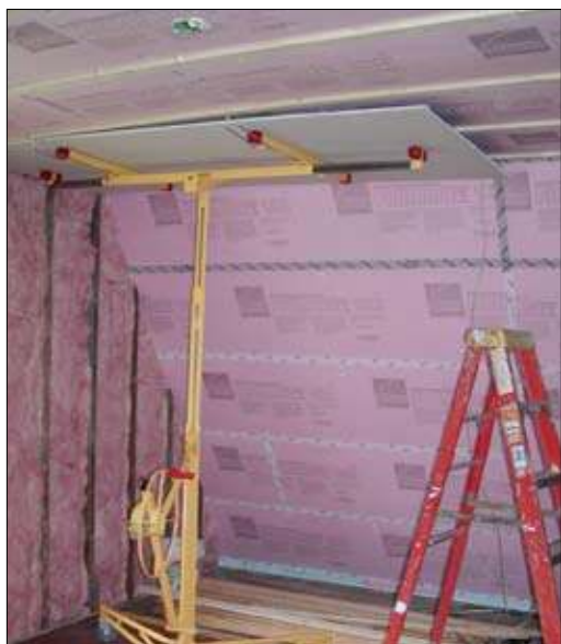
EA45 Interior Rigid Insulation and Air Seal (Taped Seams) on Ceiling
