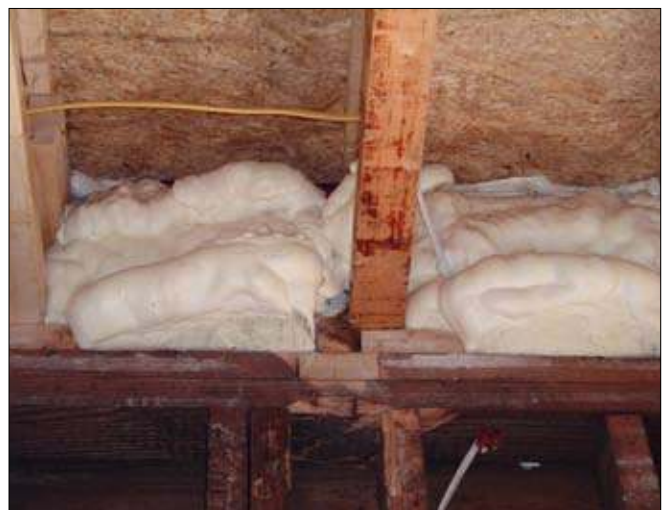
EA55 Spray-Foam Insulation at Rim Joists
