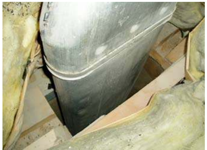
EA54 Thermal Bypass: Duct Chase
