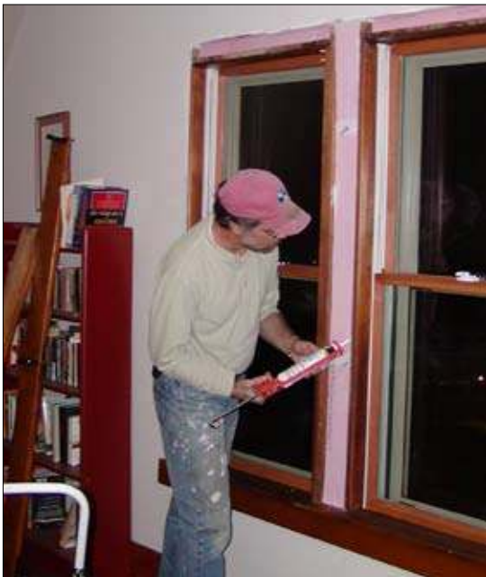
EA58 Interior Trim Removed to Insulate and Air Seal Sash Pockets after Sash Replacement
