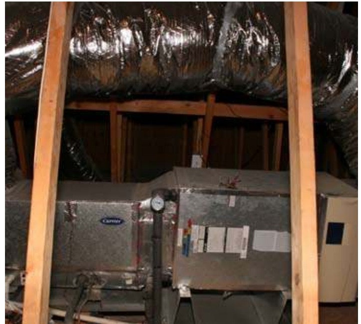
After: hydronic air handler, high-efficiency air filtration and R-6 wireflex duct work.
