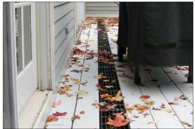
IDP25 Drip-Through Deck Grating on Gutterless Eaves
