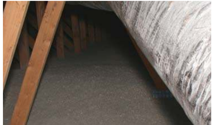
After: attic reinsulated with cellulose
