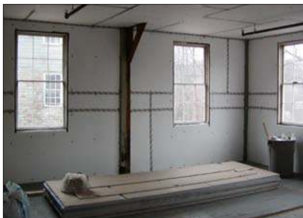
EA45 Interior Rigid Insulation (Taped Seams for Air Sealing) on Walls
