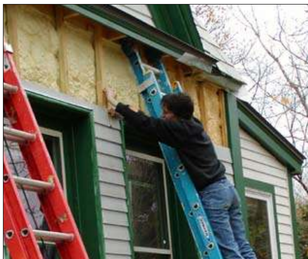
EA45 Exterior Wall Air Sealed and Insulated with Spray Foam; Reclad (Note Exterior Jamb Extensions Furring)
