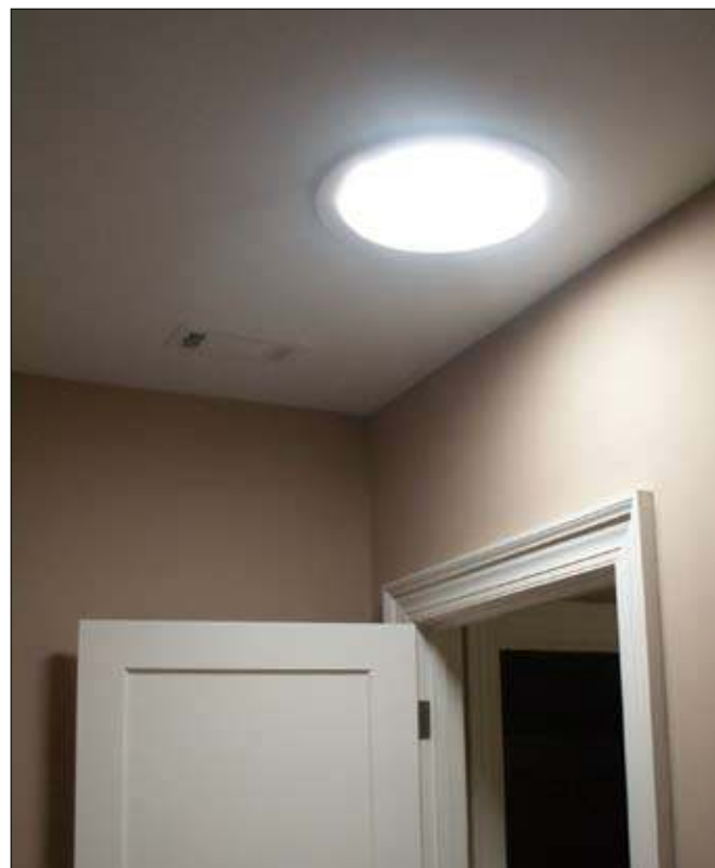
EA83 Solar Tube for Daylighting
