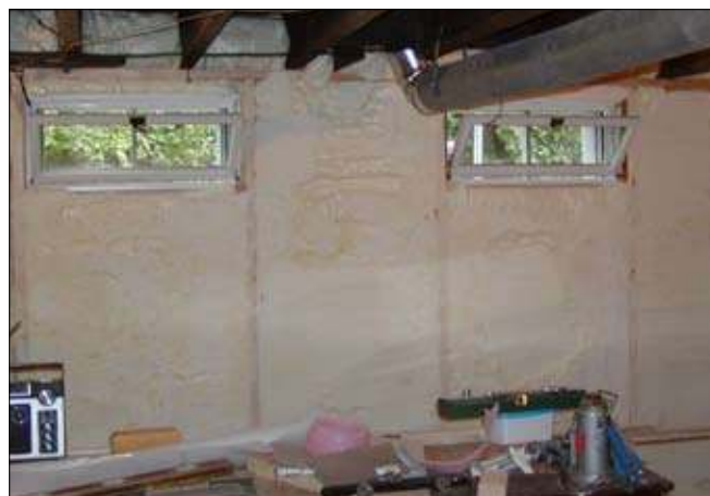
EA47 Furred-Out and Spray-Foamed Basement Walls (Vapor-Permeable Polyurethane)
