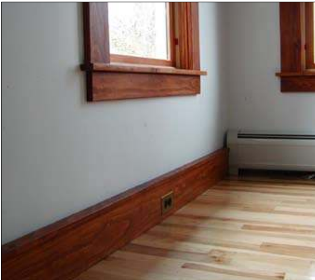
MR121 Base Board Wiring Raceway with SIP Walls
