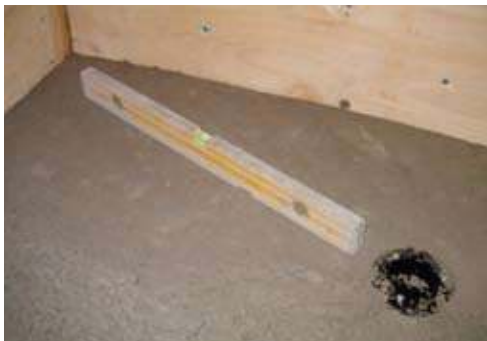
Durable shower pan, under construction
