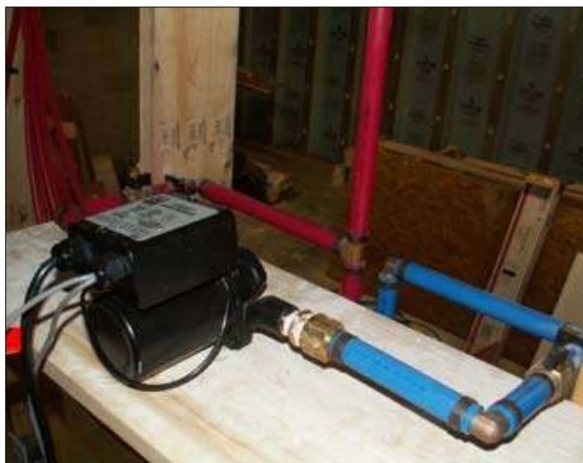
EA78 On-Demand Recirculation Pump for Hot Water
