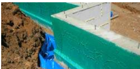
Water-managed, ICF crawlspace foundation
