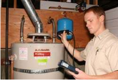
Home performance audit: testing water heater draft
