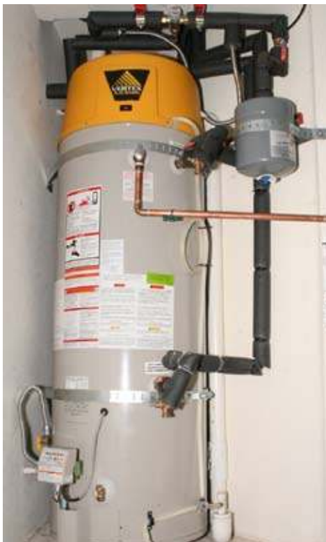
After: power-vented high-efficiency water heater
