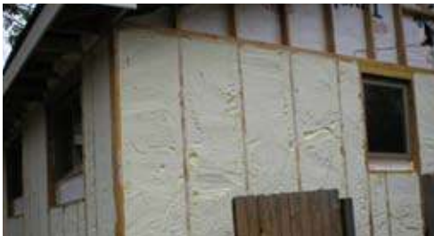
Spray foamed exterior curtain wall
