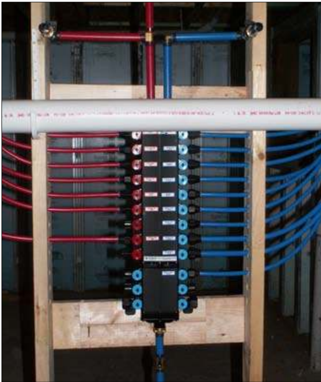
MR122 PEX Piping Manifold
