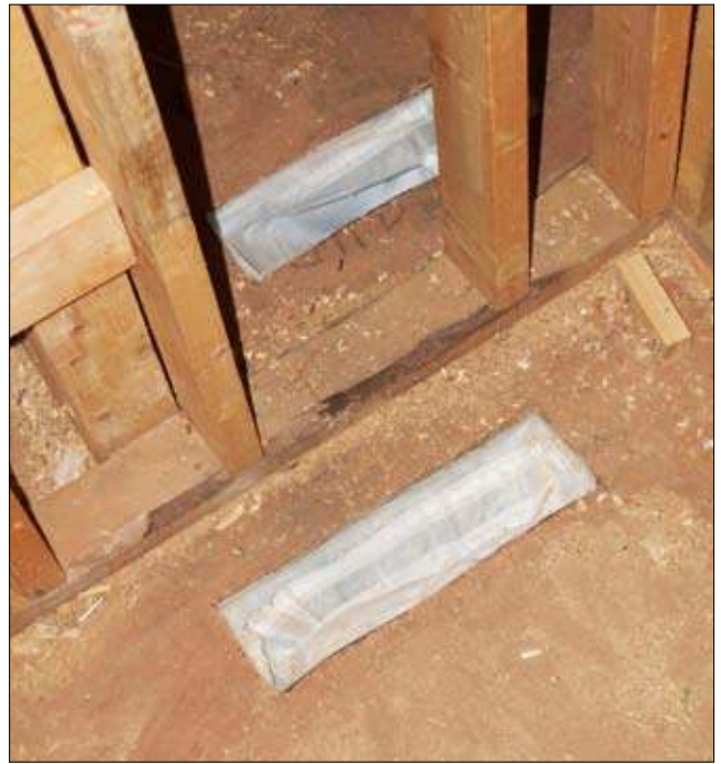
EA71 Duct Protection during Renovation
