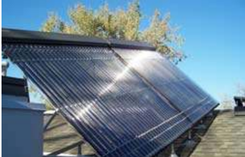
Evacuated tube solar water array
