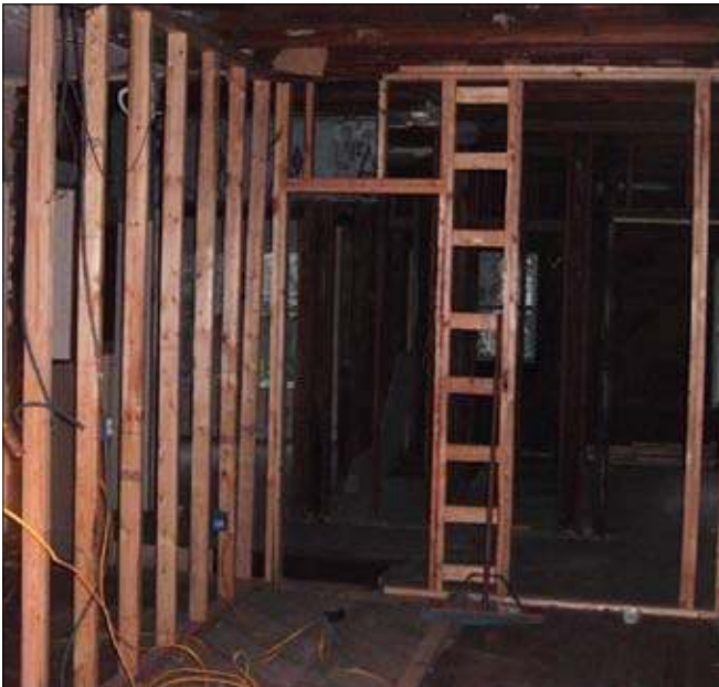
MR116 Advanced Framing on Interior Partitions
