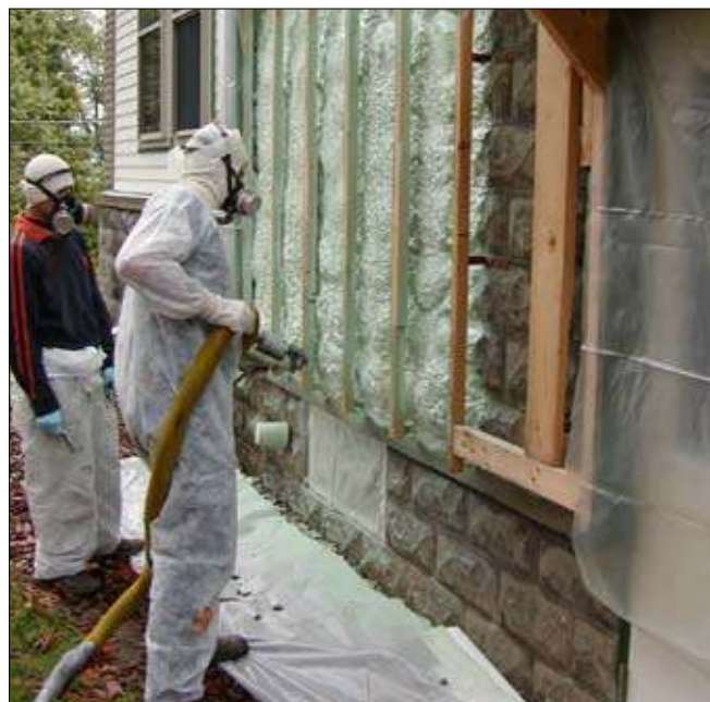
EA45 Exterior Wall Spray-Foam Insulation
