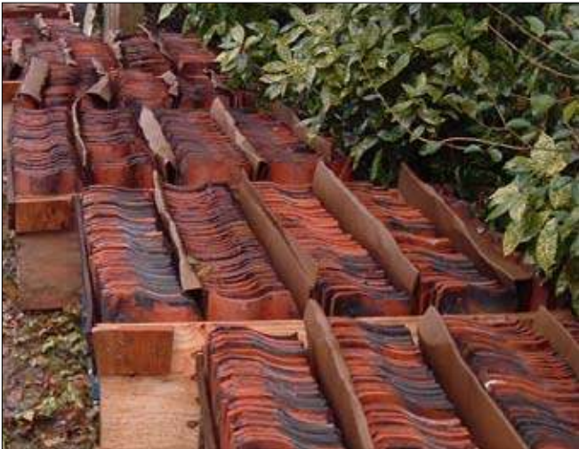
MR108 Salvaged Roofing Tiles Ready for Reinstallation
