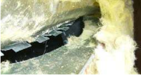
Before: duct leakage
